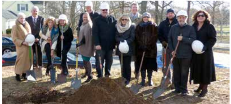
Representatives from TD Bank, Morris County Department of Human Services, Morris Township, our Project Team and HSI Executive staff assembled with hard hats and shovels for the official groundbreaking.
